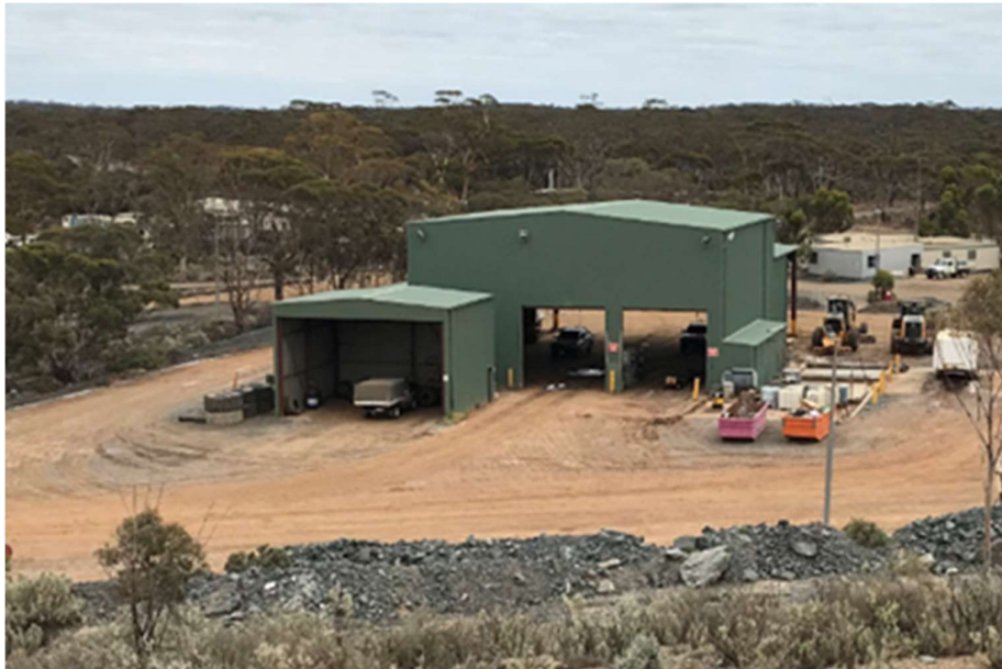
Figure 18-2 HGO underground workshop
