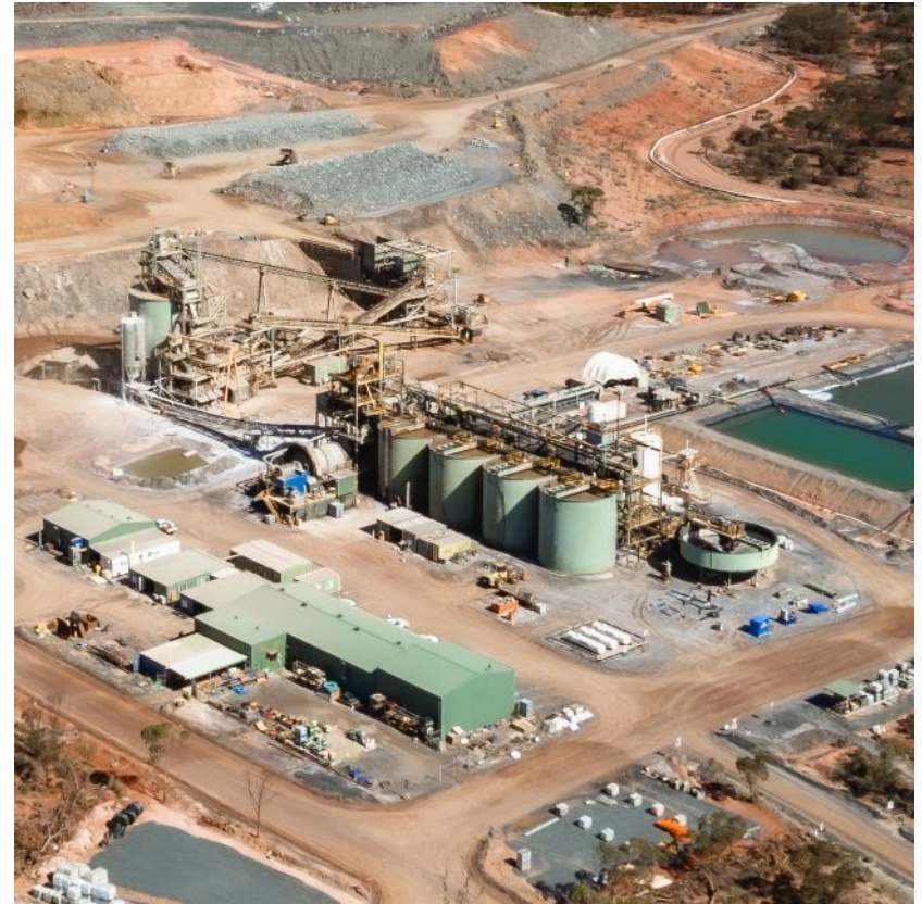
HGO Processing Plant
