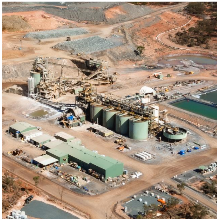
HGO Processing Plant
