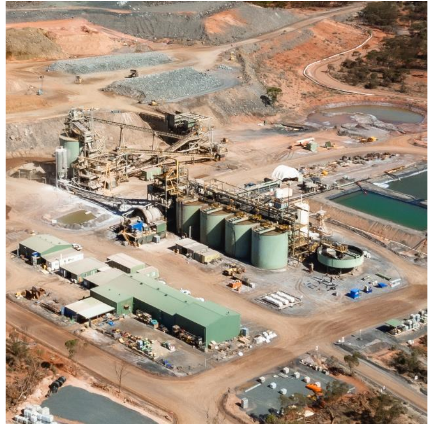
HGO Processing Plant
