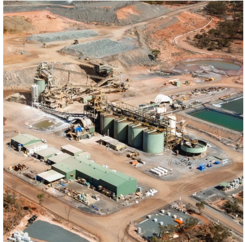
HGO Processing Plant
