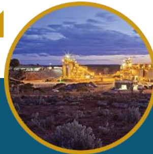
HGO mill fed at 100% capacity 1.4 Mtpa (4,000 tpd)
