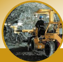
Beta Hunt Mine Underground
